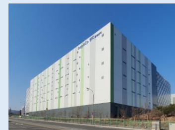
LogisCo Yangji Logistics Center
