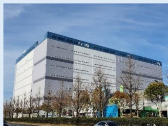
Hang-dong 7-ga Logistics Center
