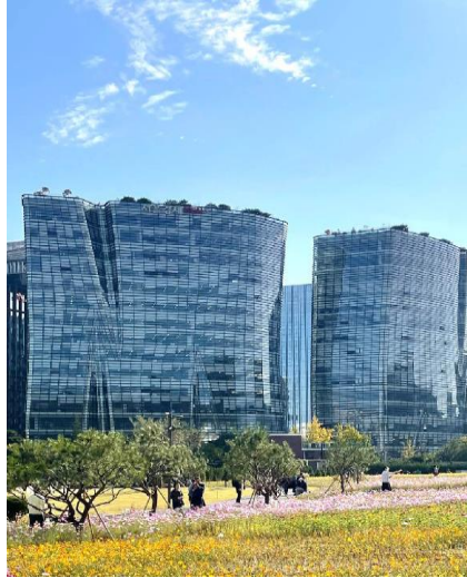
Twin Tree Tower
