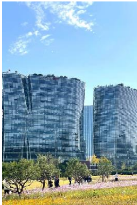
Twin Tree Tower
