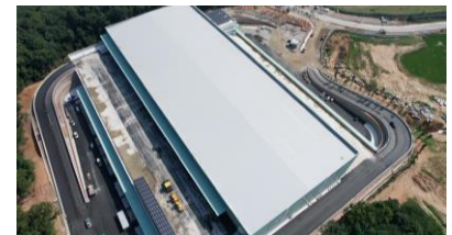
▲ Nara Logistics Center
