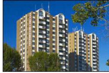
Glenmore Gardens Calgary, Alberta Rental complex 17 storey towers & garden apartments 328 units
