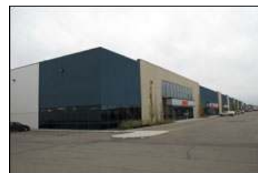
Westpoint Corporate Centre, Edmonton, Alberta Multi building industrial complex 740,000 sf
