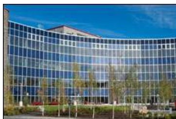
Greenstone Building Yellowknife, NW Territories Class A Downtown 4 storeys, 78,000 sf
