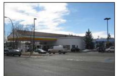
Gas Bar, Convenience store and Carwash Shell Canada Avenida Facility Calgary, Alberta 13,800 sf building on 0.95 of an acre
