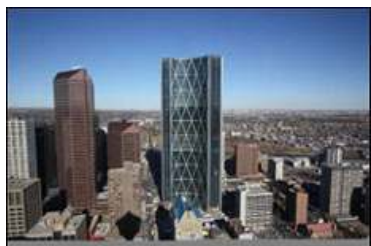
The Bow Calgary, Alberta Class AA Office 59 storeys, 2.05 million sf
