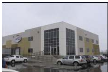
Canada Cartage Truck Terminal, Calgary, Alberta Cross dock trucking facility 30,000 sf on 13.5 acres
