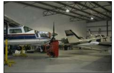
Airport Hangar Cavalier Aviation Building Springbank Airport, Alberta
