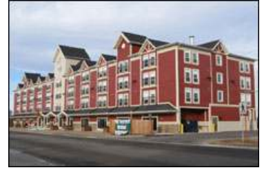
Cedar Station Airdrie, Alberta Assisted living seniors complex 87 units
