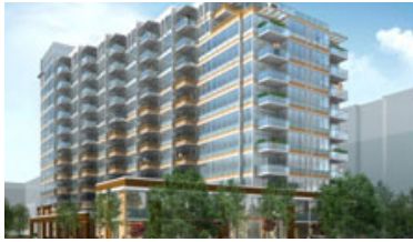
Calla Calgary, AB, New condominium building, 12 Story tower, 168 suites
