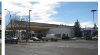
Gas Bar Shell Canada Avenida Facility Calgary, AB, 13,800 sf
