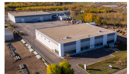
Mancal Spec Building 5804 - 51 Avenue Edmonton, AB
