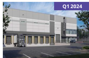
7555 Beedie Way (Leon's building expansion)
