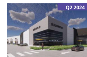
Xchange Business Park 3707 Mount Lehman Road (Building 2)
