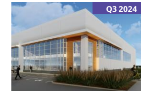
Campbell Heights Industrial Centre V 2888 194 th Street
